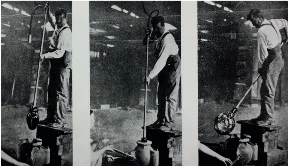
The sequence in the creation of a mold-blown glass vessel: (1). the gaffer lowers the paraison of molten glass into the mold by means of a vertical rod attached to a mechanical blowing system; (2). the mold is closed by his assistant and the glass expanded by means of compressed air pumped down the rod; (3). the completed glass vessel is removed from the mold
